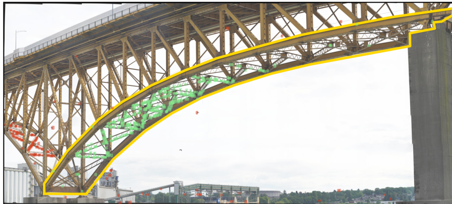
Figure 3-10: The area of the panorama that the model searches is outlined in yellow. Red boxes are detections that were excluded by this step of post-processing, and green boxes are included detections.
